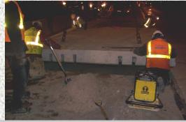
The project consisted of installation of 3 precast slabs, one in each westbound lane and the shoulder of the Reagan Memorial Tollway (I-88) to span a failed corrugated culvert. The emergency repair was intended to be in place for approximately one year until that section of the Tollway was reconstructed as part of a major bridge and roadway reconstruction project.
